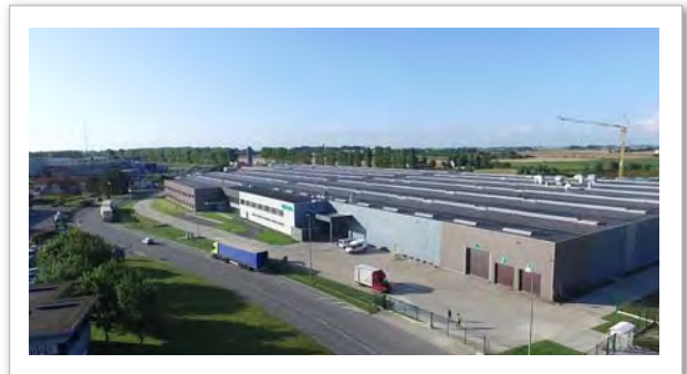
▲ Aerial view of KFM.
