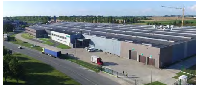
Aerial view of KFM.
